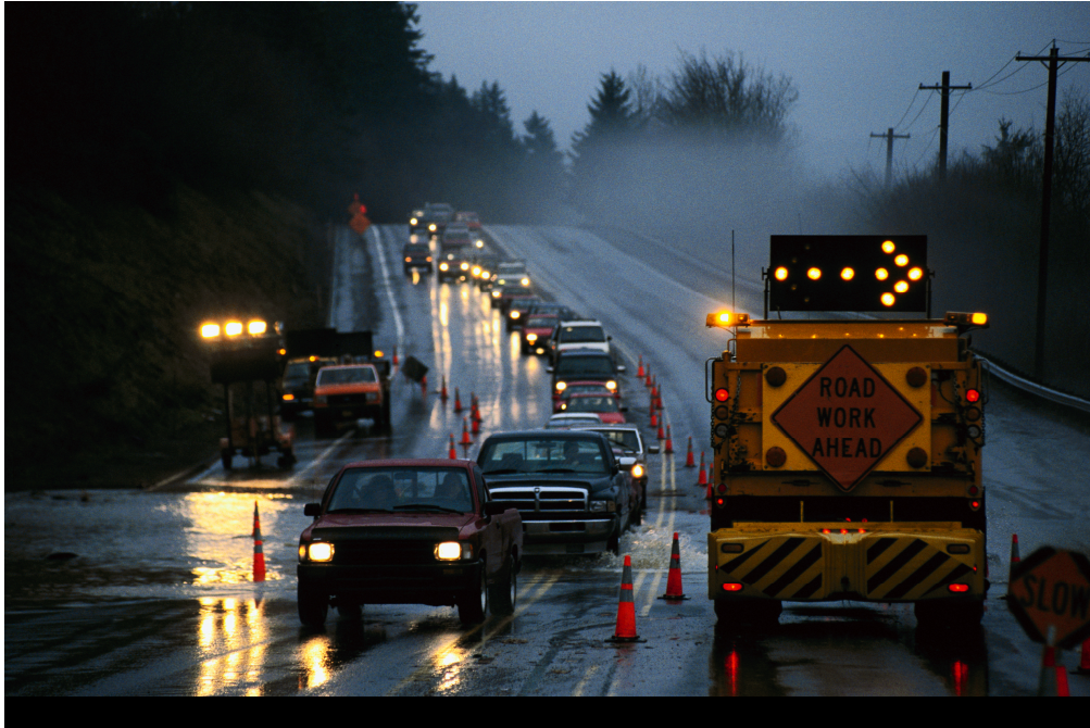
Figure 3.6 Project Open to Traffic (Source: MyConstructionPhotos)
