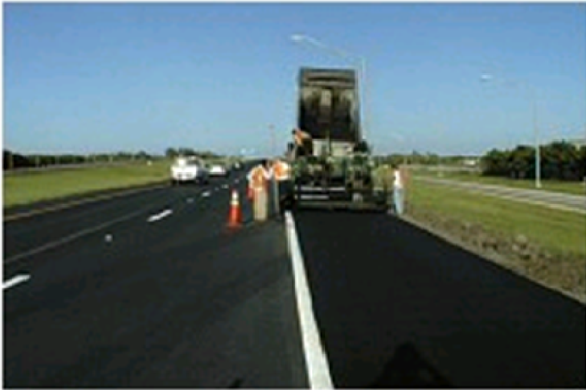
Figure 3.4 HMA Project (Source: MyConstructionPhotos)
